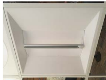
Figures – Cree 2x2 LED troffer directly connected via RJ45 (Source: MN CEE)
