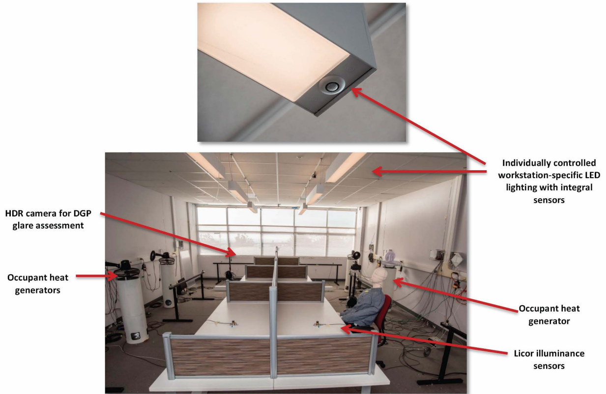
Figure 10: FLEXLAB Internal Test Cell View with Key Features
