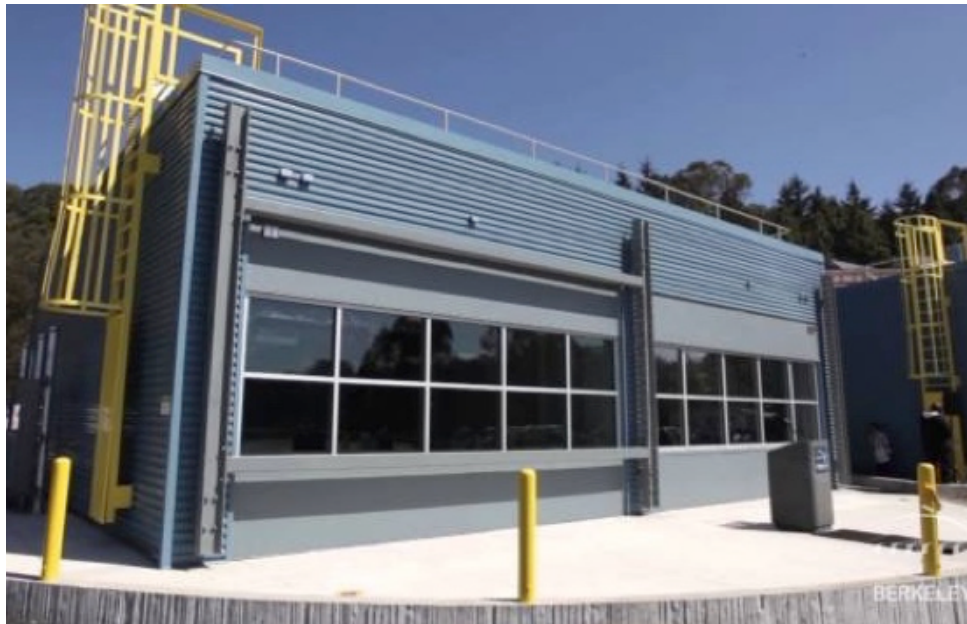
Figure 2. External view of the FLEXLAB rotating testbed
