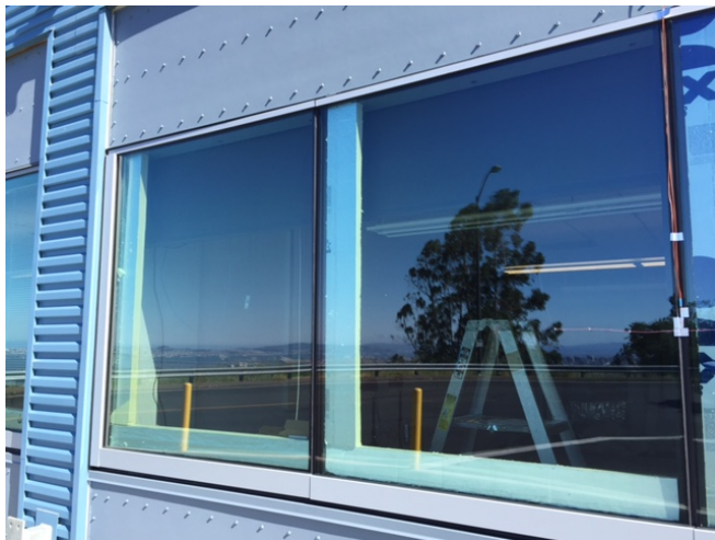
9 Paneling for lower window-to-wall ratio
