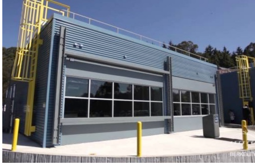
Figure 3. External view of the FLEXLAB rotating testbed
