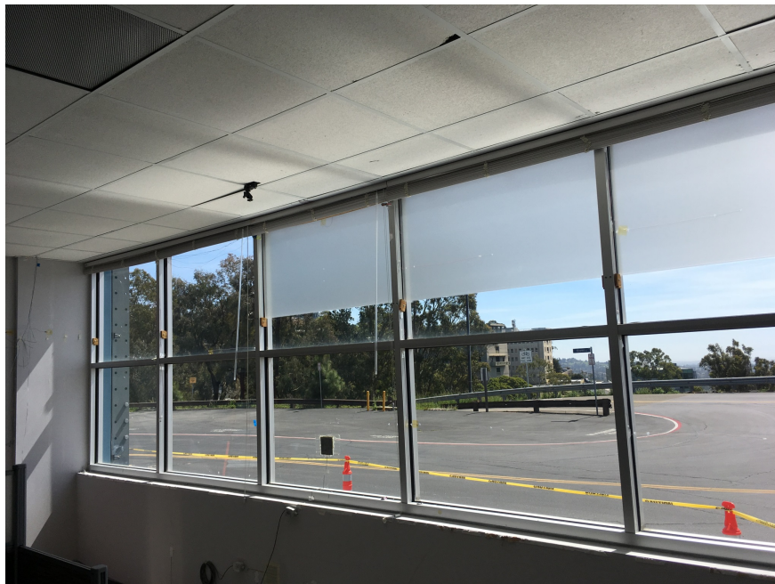
Figure D-1: Film 2 Installed in Upper Right Window Panes
